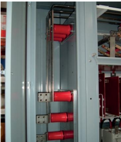
Figure 5.4 Incoming Power Termination Bus System
